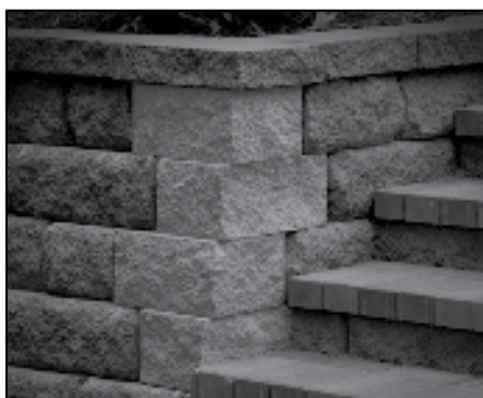
Outside 90-Degree Corner with Corner/Column Unit
