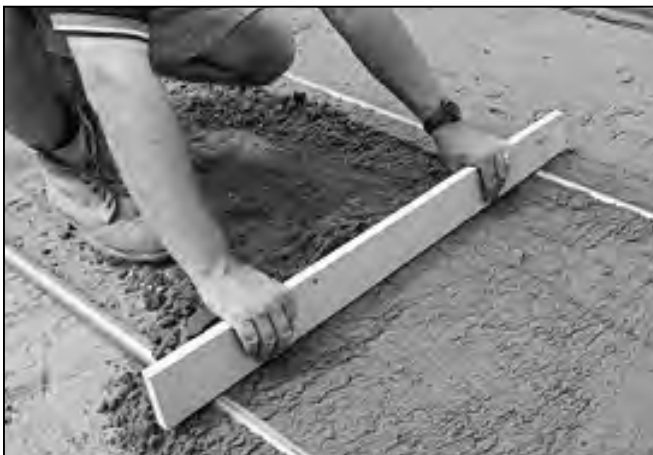
Install bedding sand.
