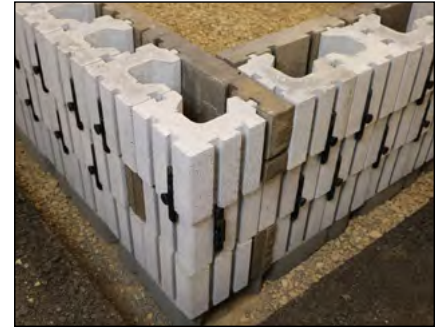
Diagram 12—Corner unit formed
