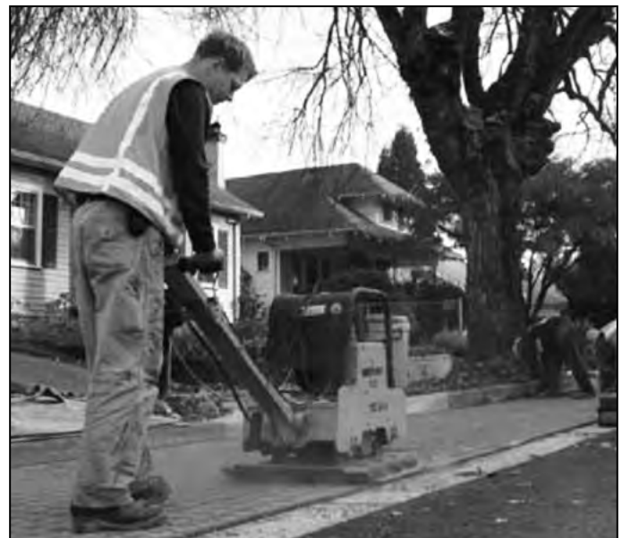
PICP paver compaction shows that pavers need to be set about \frac{3}{4} -inch (19 mm) above their final elevation before compaction and \frac{3}{8} -inch (10 mm) after compaction to account for downward movement.
