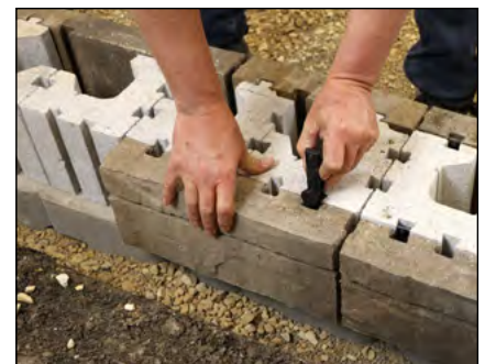
Diagram 20—Placing veneers onto modular block
