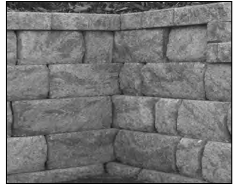
Example Inside 90-Degree Corner
