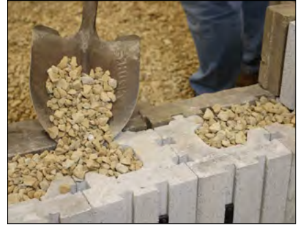
Diagram 5—Fill cores with free draining aggregate
