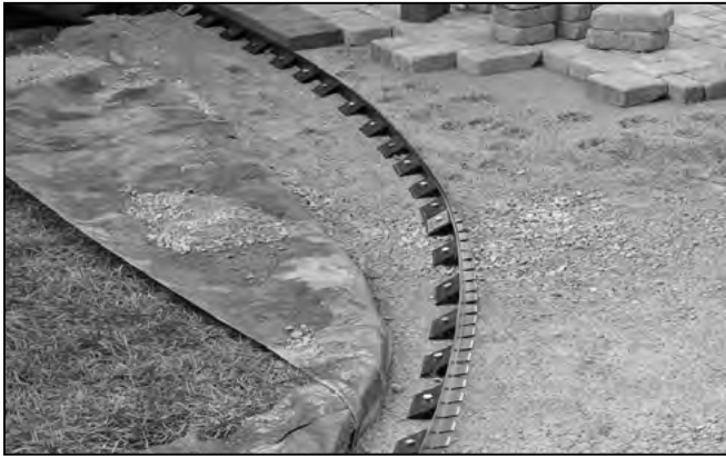
Install edge restraints.
