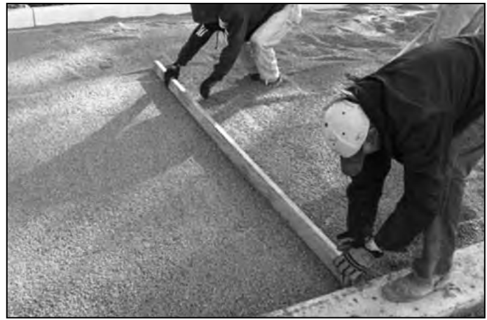
Manually screeding the No. 8 stone setting bed.
