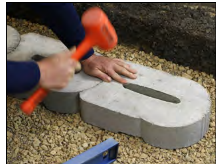
Diagram 3—Lay and level base block
