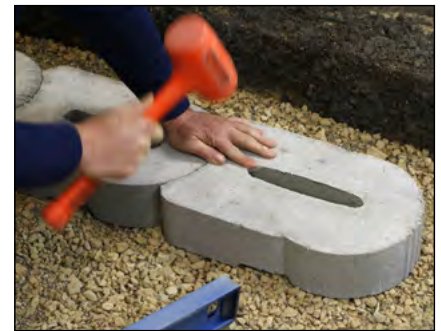
Diagram 19—Lay and level base block
