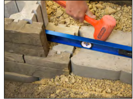
Diagram 7—Stepping up the base
