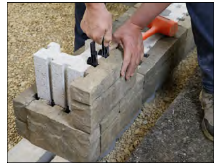
Diagram 22—Wall end example
