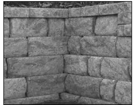
Example Inside 90-Degree Corner
