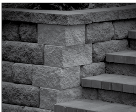
Outside 90-Degree Corner with Corner/Column Unit
