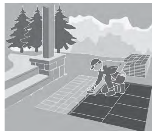
STEP 6: INSTALL PAVERS
