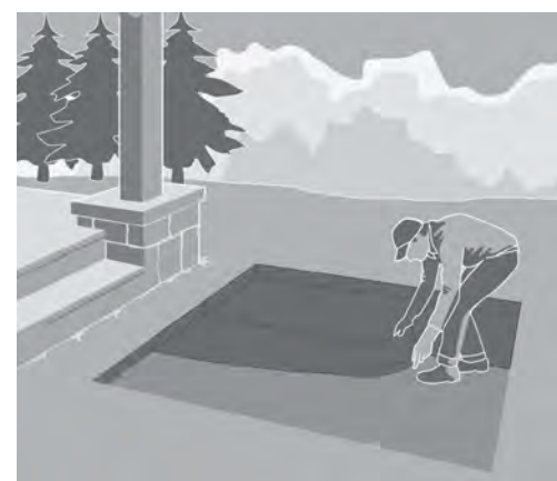
STEP 3: LAY GEOTEXTILE
